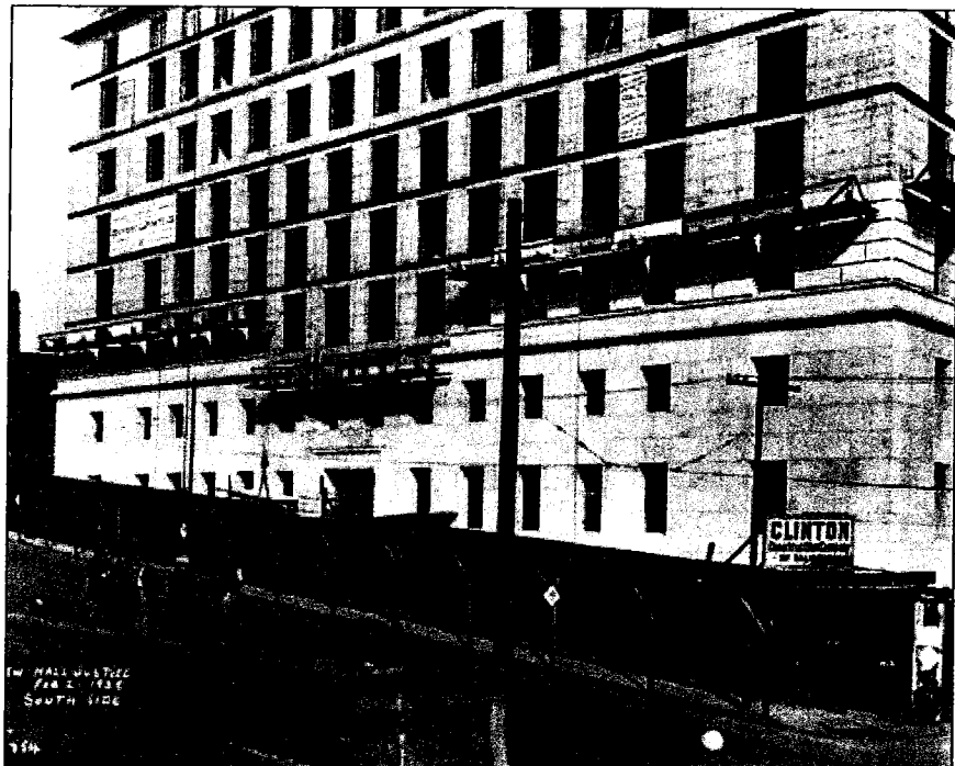
Photo 5: Installing granite on the south side of the Hall of Justice, 1925. Temple Street (south) façade, looking north. (Los Angeles Public Library Photo Database)
