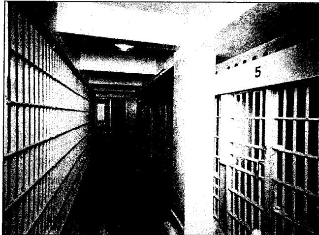
Figure 3: Typical jail corridor with double row of steel bars. (Los Angeles Public Library Photo Database)
