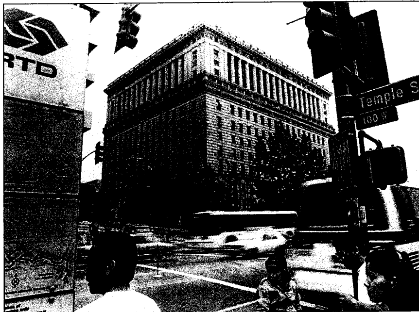
Photo 29: Hall of Justice, 1982. Temple and Spring Streets, looking northwest. (Los Angeles Public Library Photo Database)
