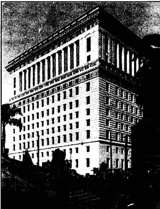
Figure 6: The Hall of Justice in 1934. The tripartite division of the each façade is a distinct visual characteristic of the building. (Los Angeles Public Library Photo Database)
