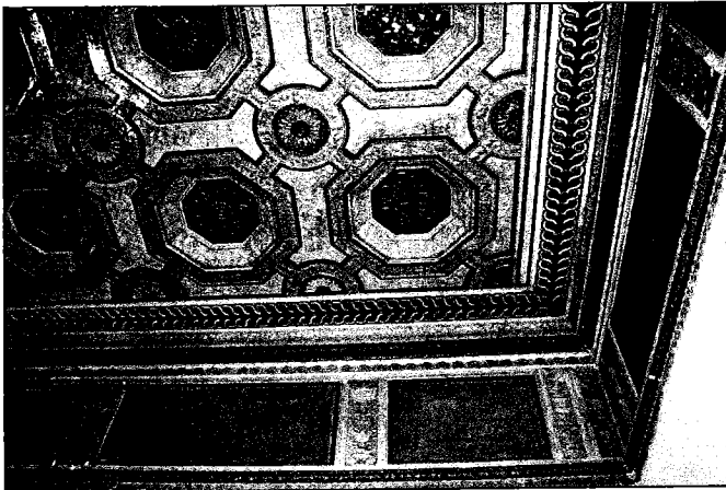
Figure 14: Ornamental plaster ceiling in courtroom, 2001. (Historic Resources Group)
