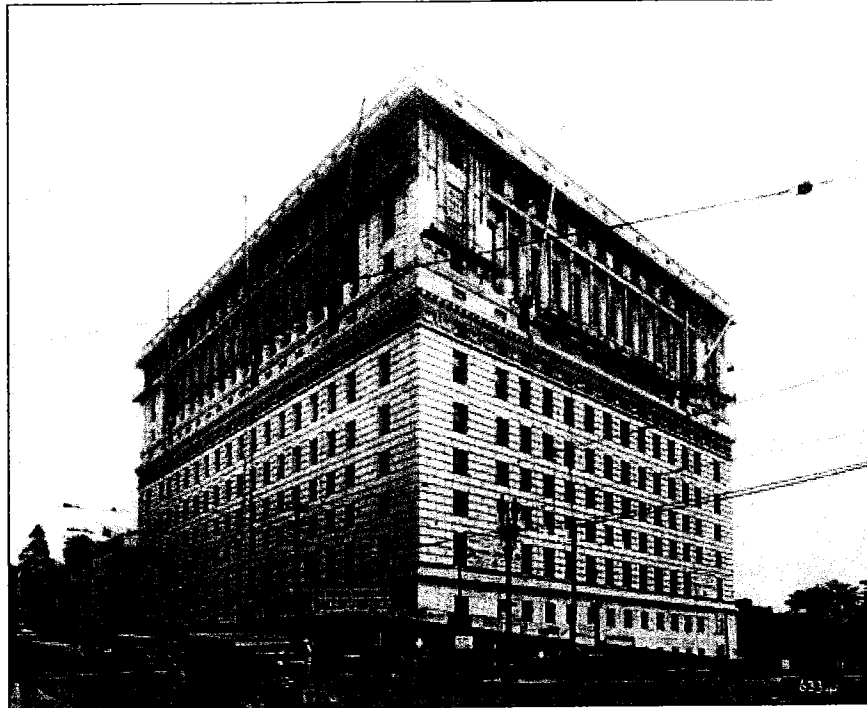
Photo 6: Construction of the Hall of Justice nearing completion, 1925. Broadway and Temple Street, looking northwest. (Los Angeles Public Library Photo Database)
