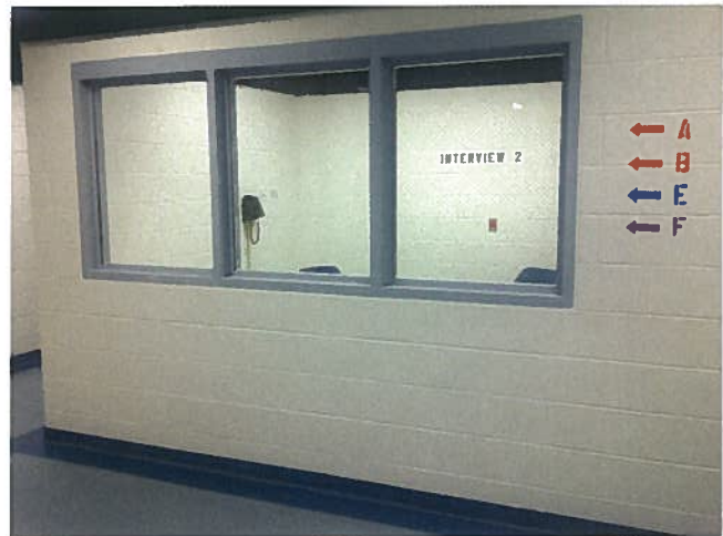
DETENTION FACILITY – Contact Visitation Room
