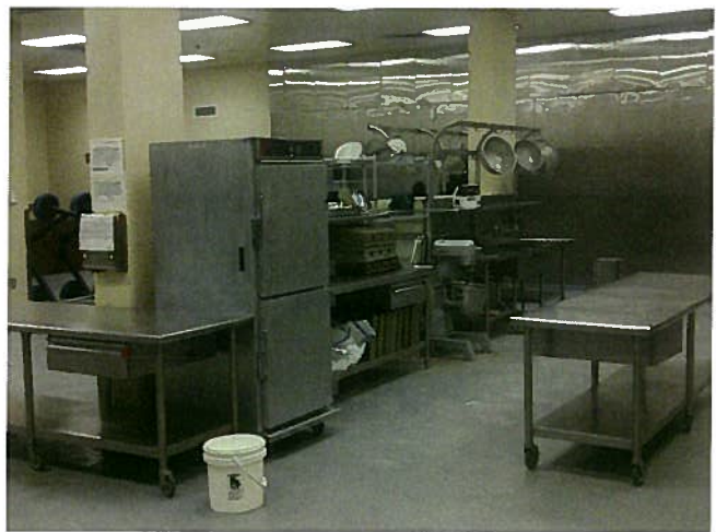
DETENTION FACILITY – Food Services Facility
