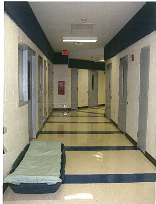
DETENTION FACILITY – Corridors
