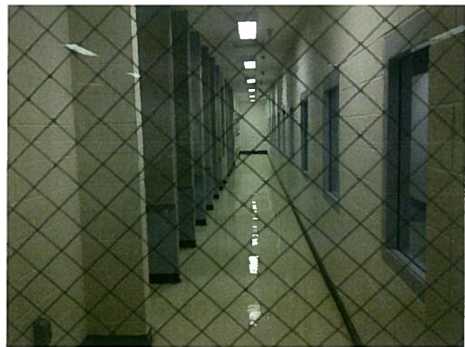
DETENTION FACILITY – Visitor's Side, Old Visitation Center
