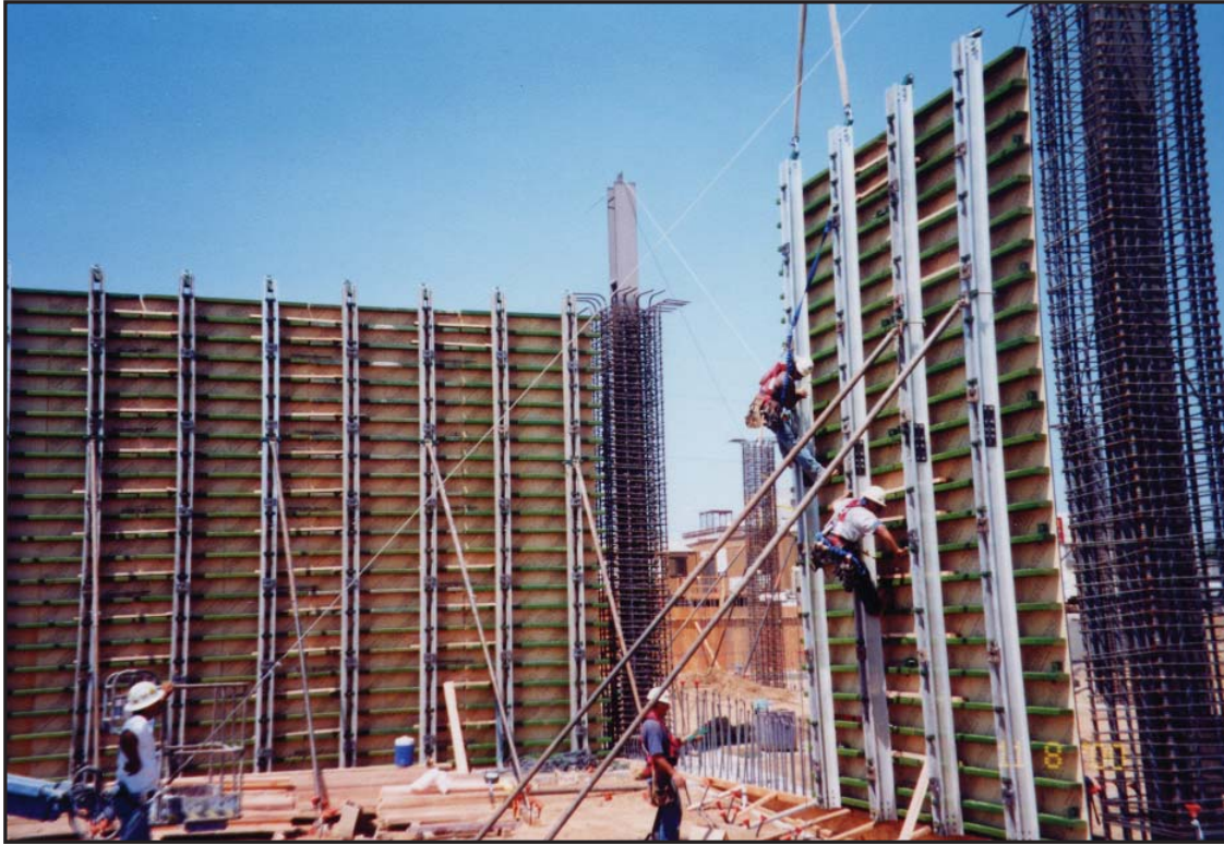
8' X 25' FORMS FABRICATED OFFSITE AND SHIPPED READY FOR FINISHED PLACEMENT
