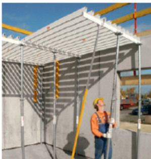
... mount prop and position vertically.
