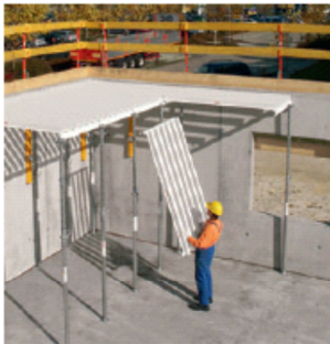
Hook in GRIDFLEX element at one end ...
