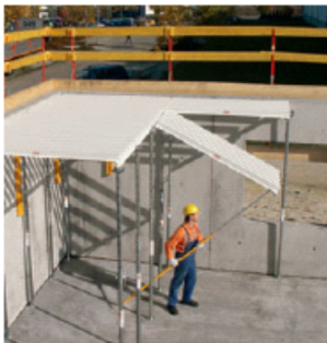
... align horizontally with the shuttering aid ...
