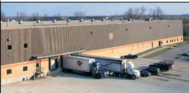
Link-Belt Parts Distribution Center
