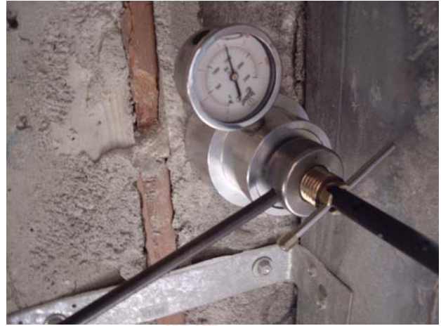
Testing the Granite Veneer
