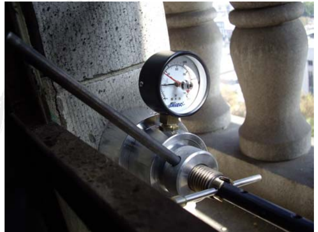
Testing the Terra Cotta Veneer
