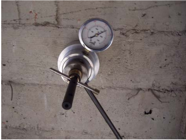
Testing the Poured Concrete Back-up
