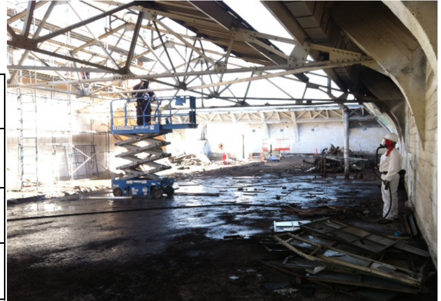
Demo Workers donned in full protective gear
