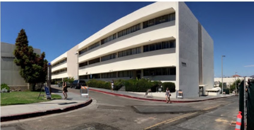
d view of existing engineering building
