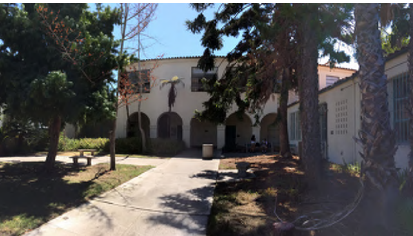
e view of existing courtyard
