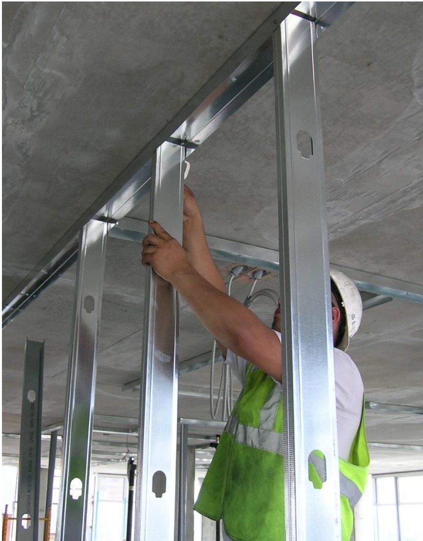
ViperStud® Drywall Framing being installed on a jobsite.
