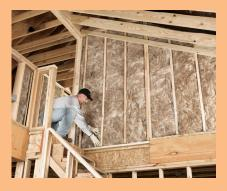
**EcoBatt insulation is naturally brown**– ensures no phenol, formaldehyde, acrylics or artificial colors are used in the manufacturing process.
