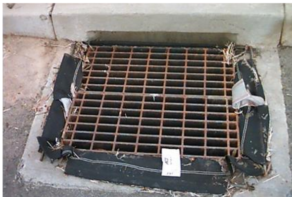
Catch Basin Insert Bag No overflow and normal flow only
