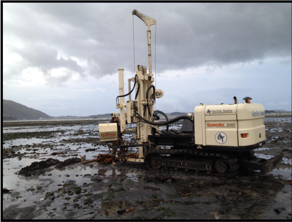
Drill rig set up on TH 12-08
