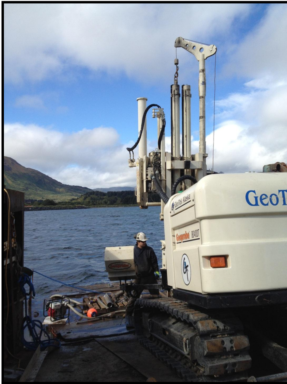
8040 on landing craft drilling TH12-07
