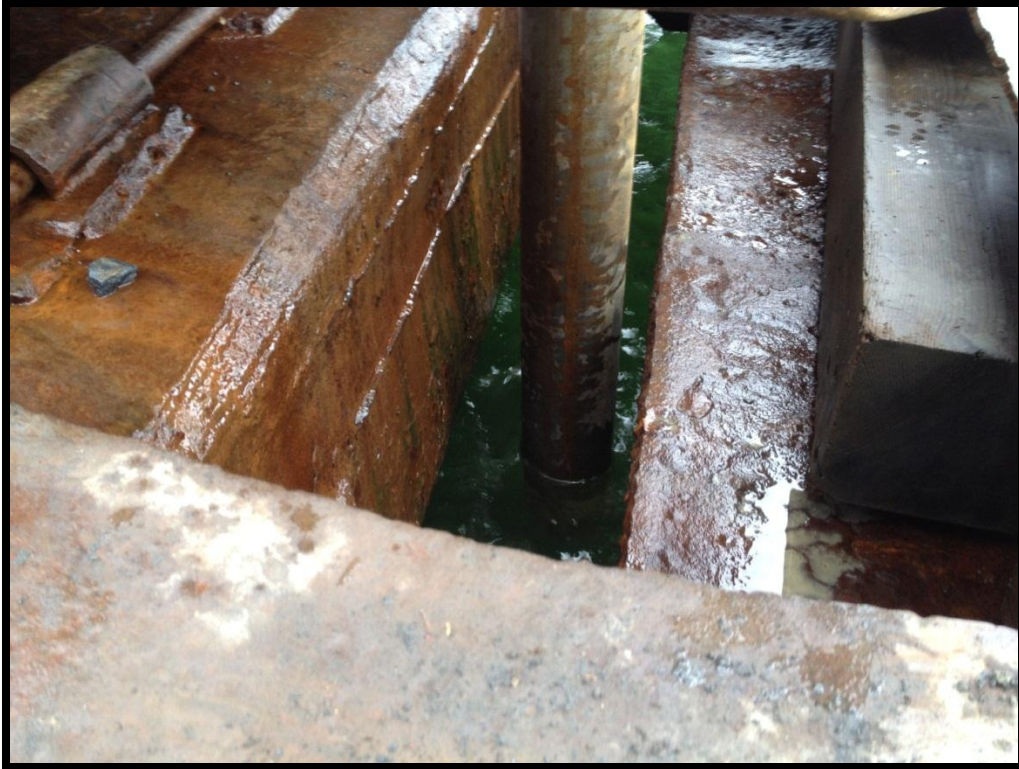
Casing in hole on landingcraft
