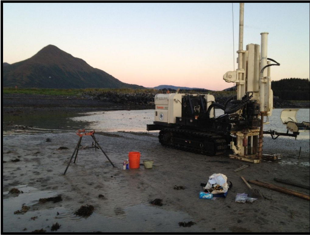
Drill rig set up on TH 12-04
