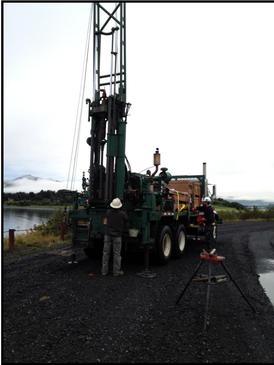
Drill rig set up on TH12-02
