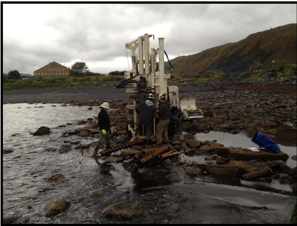
Drill rig set up on TH12-09
