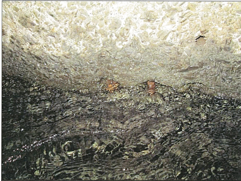
PHOTO 3: LOWER EAST WALL OF WEST BAY AT STATION 90.
