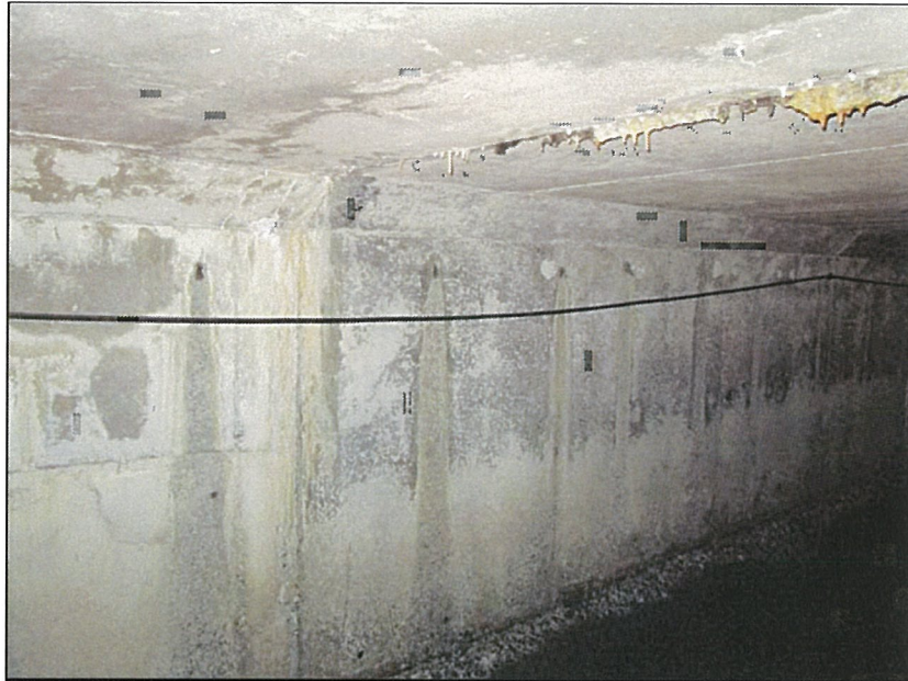
PHOTO 19: EAST WALL OF EAST BAY AT STATION 240.
