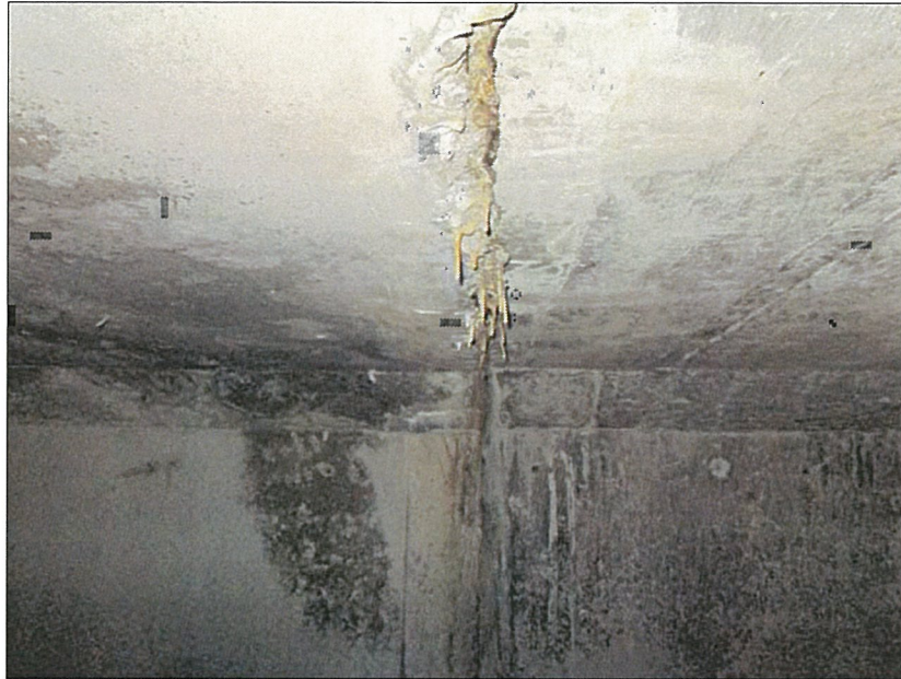
PHOTO 5: LOOKING EAST AT CEILING OF WEST BAY AT STATION 240.
