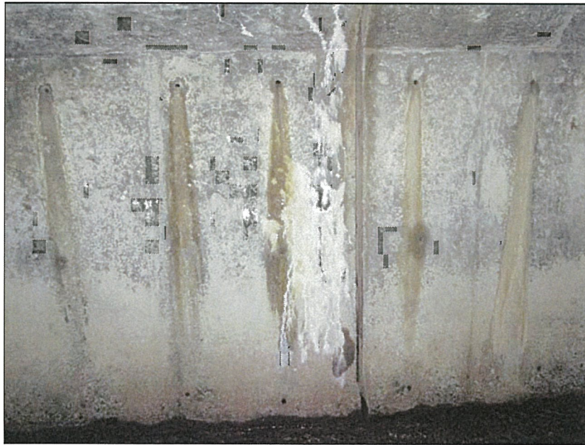
PHOTO 4: WEST WALL OF WEST BAY AT STATION 1955.
