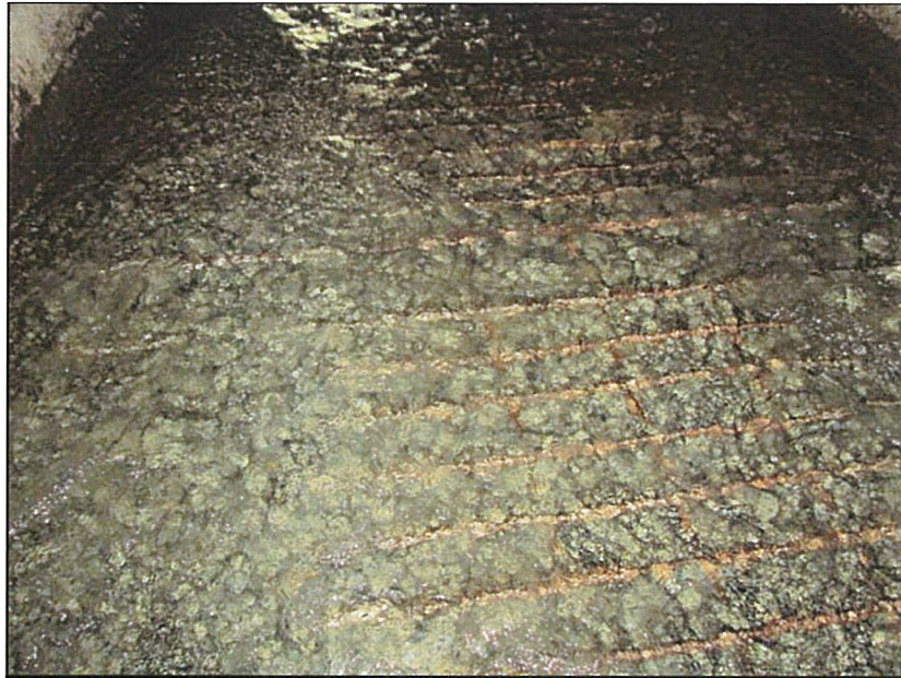
PHOTO 11: FLOOR OF WEST BAY AT STATION 685.
