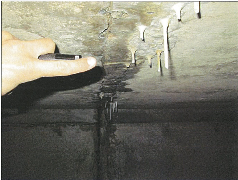
PHOTO 8: LOOKING WEST AT CEILING OF WEST BAY AT STATION 465.
