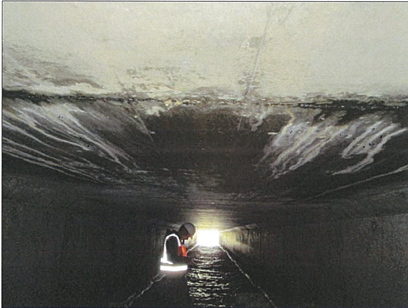
PHOTO 10: CENTER OF CEILING OF WEST BAY AT STATION 620.
