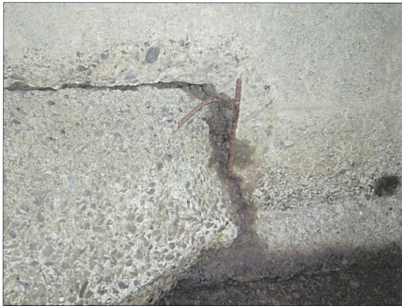
PHOTO 22: LOWER EAST WALL OF EAST BAY AT STATION 420.
