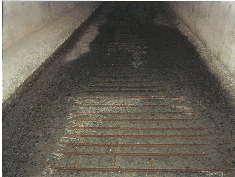
PHOTO 23: FLOOR OF EAST BAY AT STATION 605.
