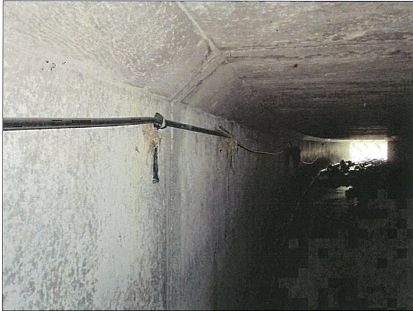
PHOTO 15: EAST WALL OF EAST BAY AT STATION 90.
