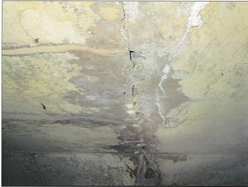
PHOTO 9: LOOKING EAST AT CEILING OF WEST BAY AT STATION 495.
