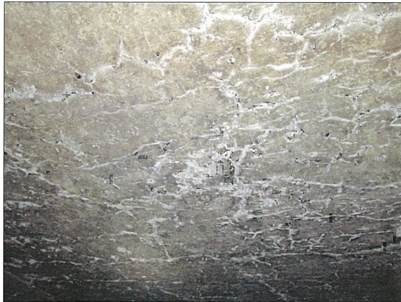
PHOTO 17: CENTER OF CEILING OF EAST BAY AT STATION 145.
