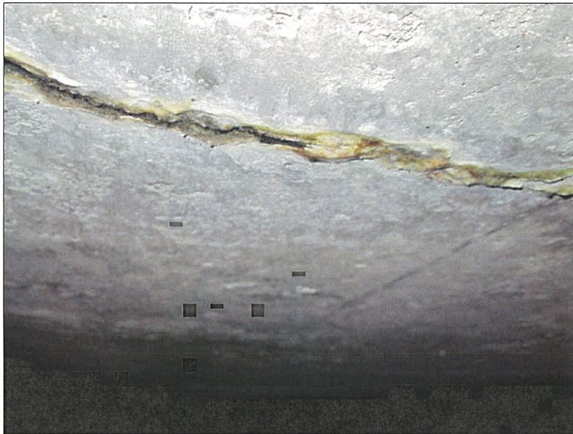
PHOTO 26: CENTER OF CEILING OF EAST BAY AT STATION 745.
