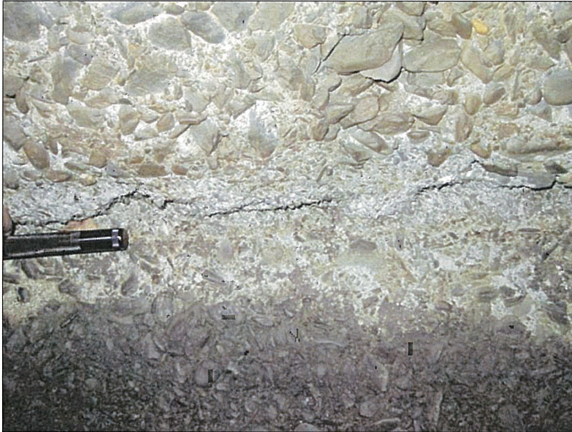
PHOTO 16: LOWER EAST WALL OF EAST BAY AT STATION 115.
