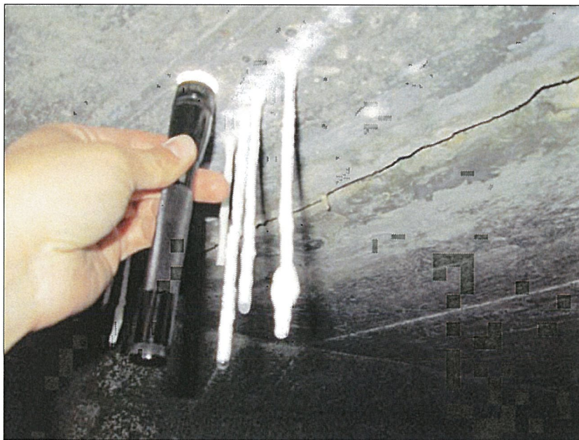
PHOTO 18: LOOKING WEST AT CEILING OF EAST BAY AT STATION 150.
