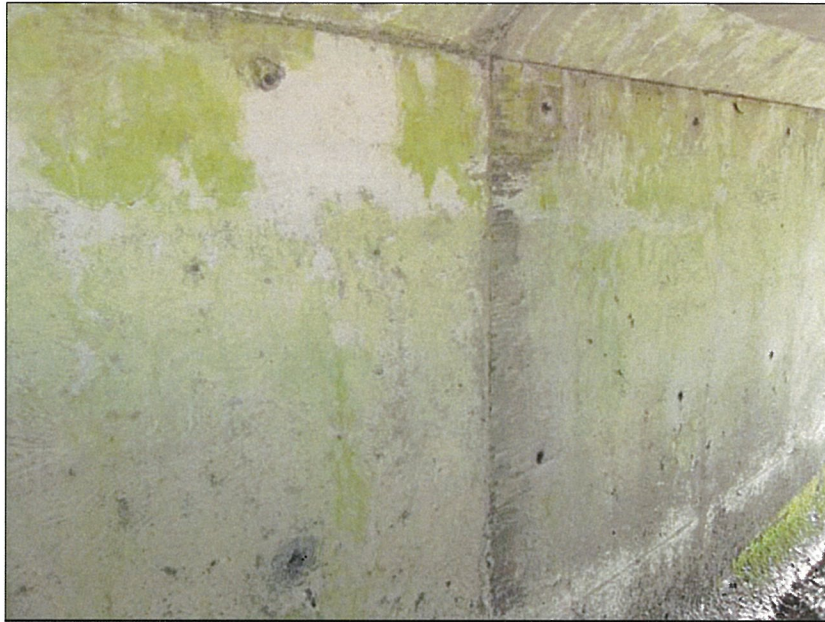
PHOTO 13: WEST WALL OF WEST BAY AT STATION 770.
