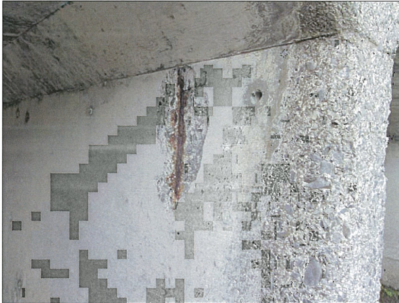
PHOTO 2: TOP OF CENTER WALL AT CULVERT INLET.
