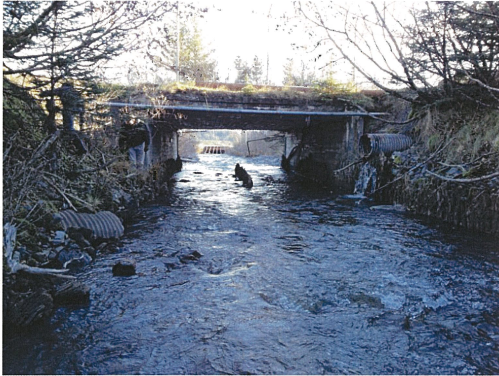
Maintenance road bridge—note airport culvert intake in background.
