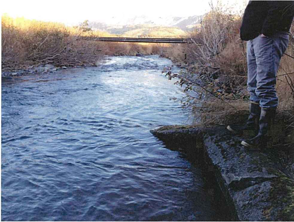
Tailwater section for airport culvert outlet. Photograph looking downstream
