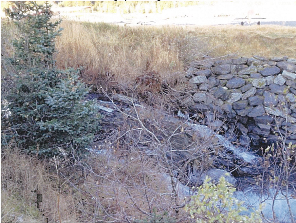
Waterfall downstream of airport culvert outlet.
