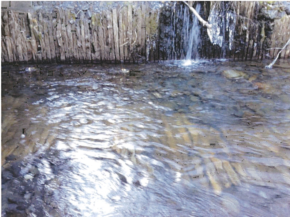
Relic wooden box culvert; detail of timber bottom.
