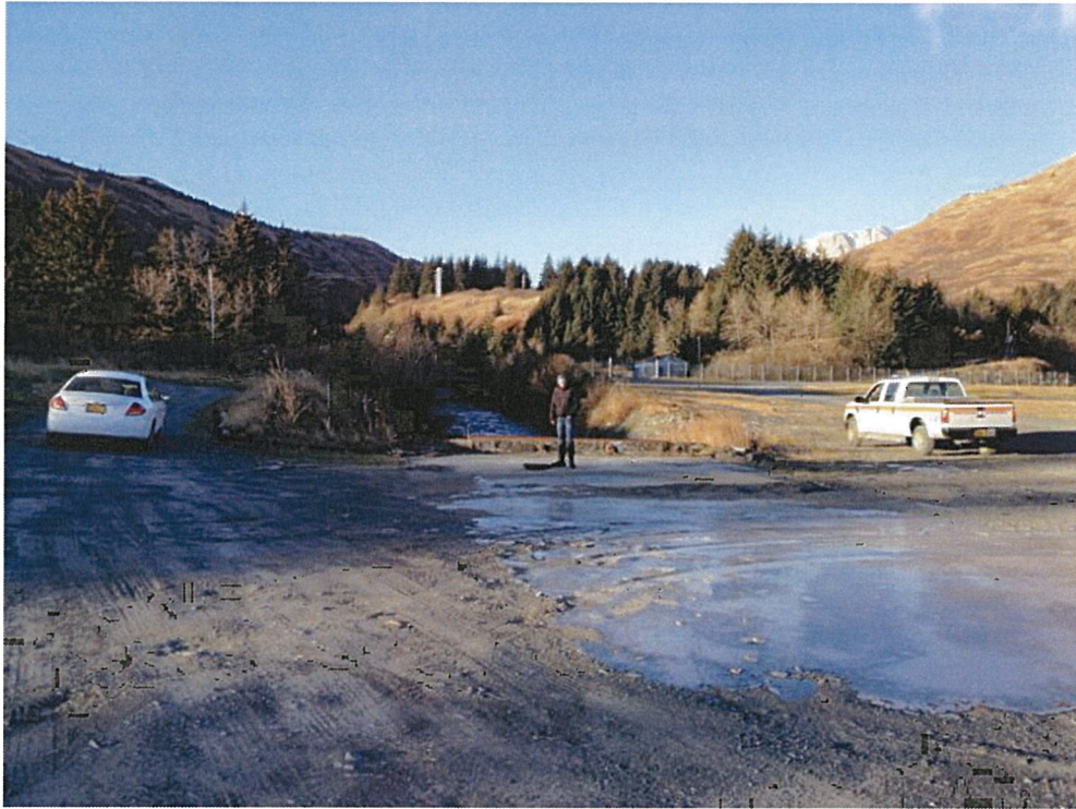
Airport culvert intake Photograph looking upstream
