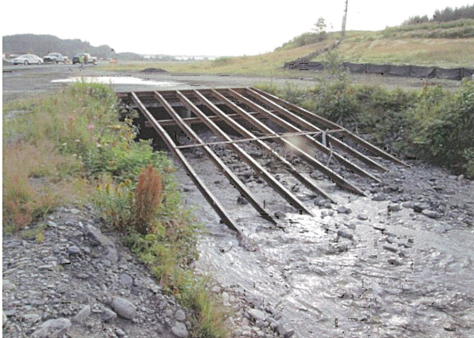
Airport culvert intake and debris rack. Photograph looking downstream.
