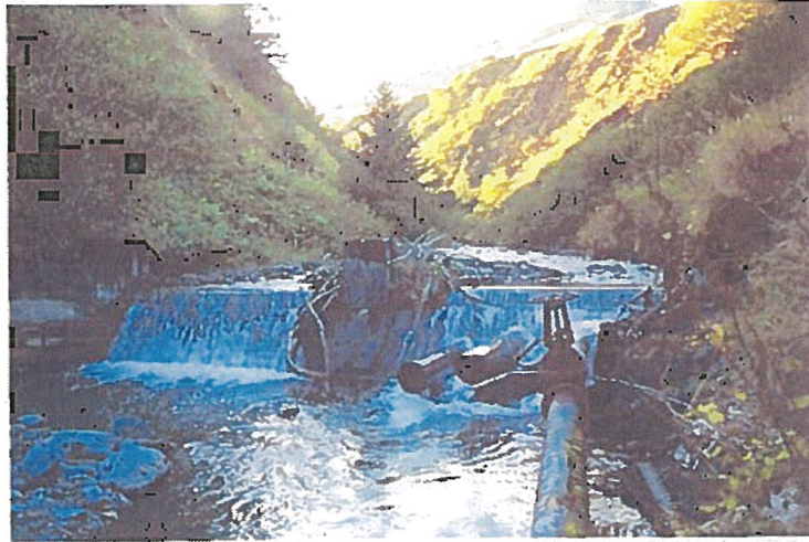
FIGURE 29. Weir on Devils Creek (Photo by others)
