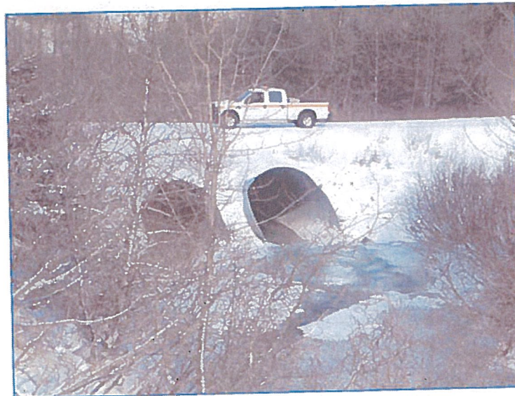
FIGURE 20. Culverts beneath an access road, downstream of the concrete box culvert.
