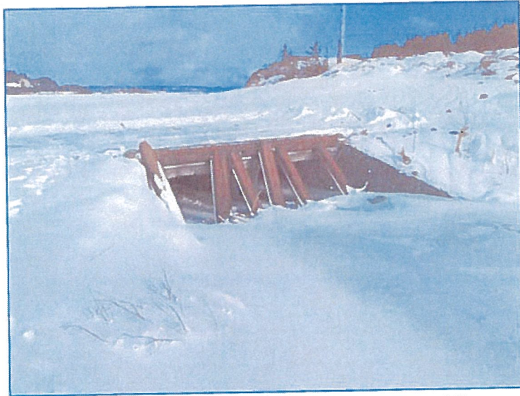
FIGURE 1. Culvert inlet and “debris rack”.
