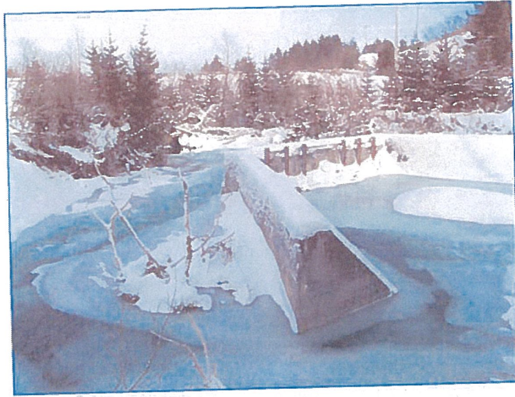
FIGURE 25. Another view of the concrete structure upstream of Rezanof Drive.
