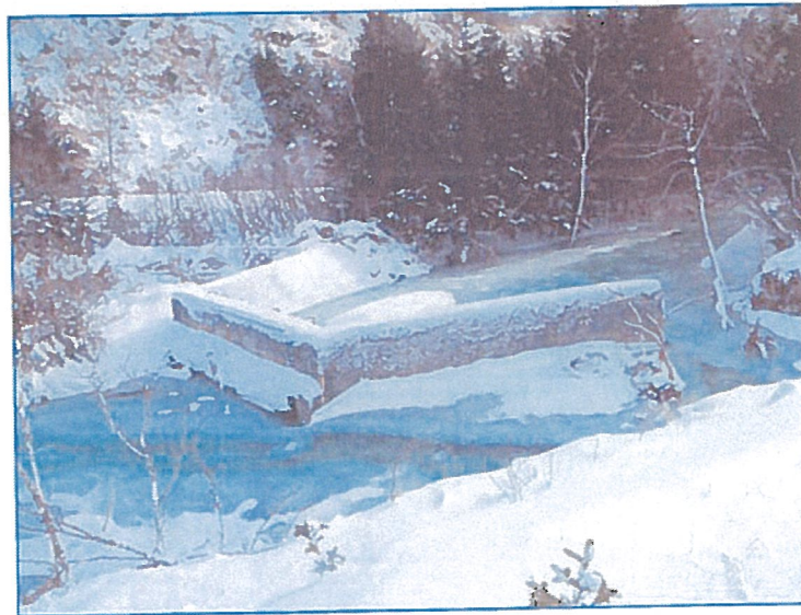
FIGURE 24. A concrete structure upstream of Rezanof Drive.
