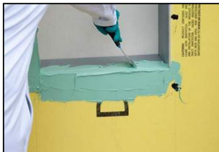
Figure 1: Application of Dow Corning 778 Liquid Flashing.
