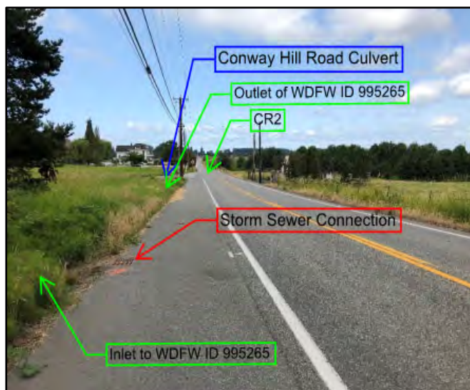
Figure 2.7. Layout of the Barrier WDFW ID 995265 (looking west down SR 534)
