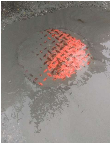
EXHIBIT 2-2. WATER FLOWING ABOVE THE GROUND SURFACE DURING BOREHOLE SEALING
