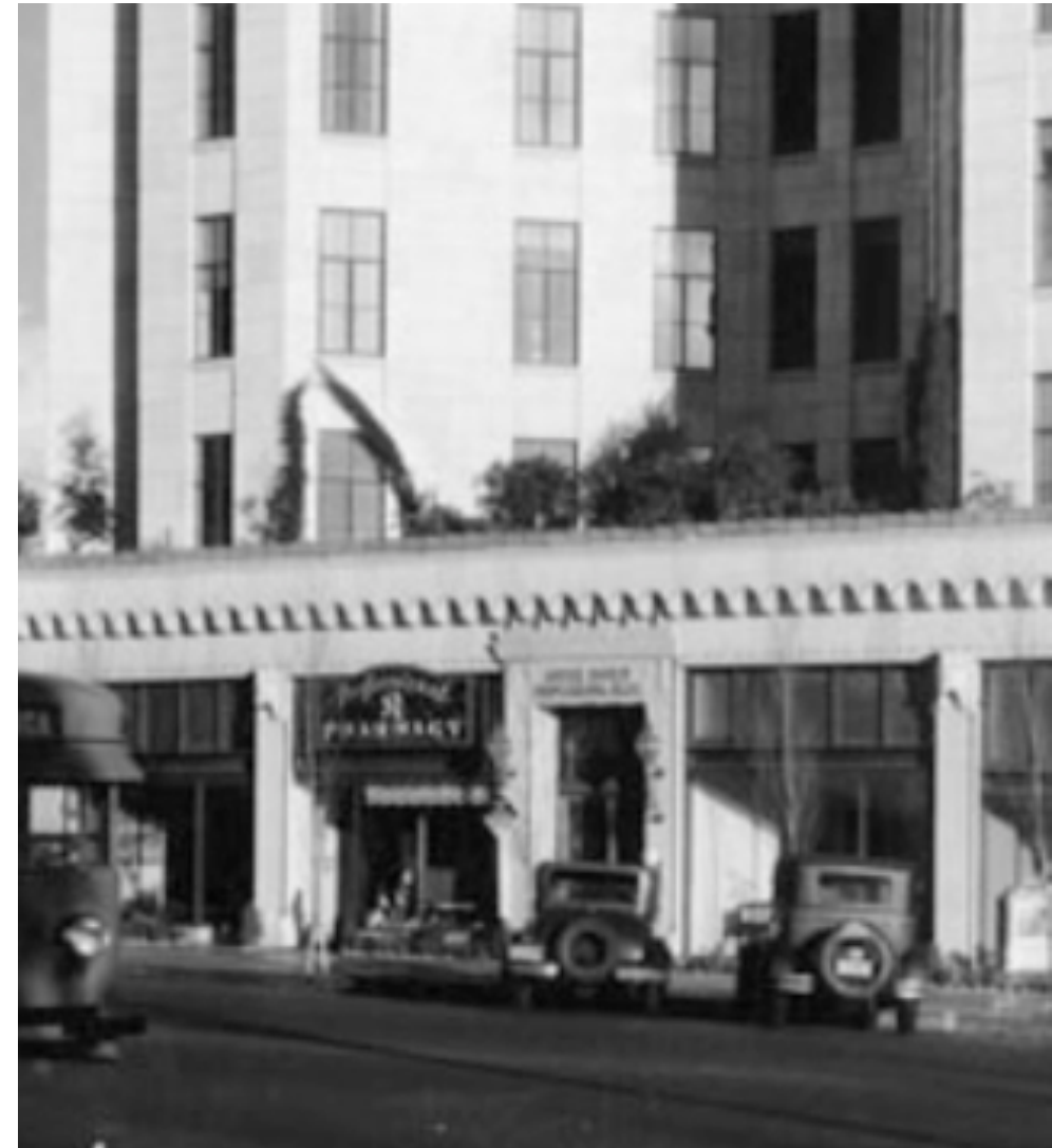
Detail. The parapet, as well as the faux ashlar walls, exhibit tonal variations of individual "blocks". A finish coat of white stucco matrix with fine sand may be the first layer in contact with the cast concrete. This may have been subtly tinted or textured for aesthetic effect to enhance the illusion of natural stone.
