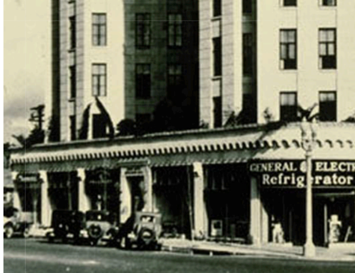
Santa Monica Professional Building, 710 Wilshire Blvd. Note the subtle tonal variations in the faux ashlar blocks, most apparent in the shadow at upper left of center, appear slightly more pronounced than the slightly earlier photos. Differential soiling or moisture retention may already be enhancing the differences.
