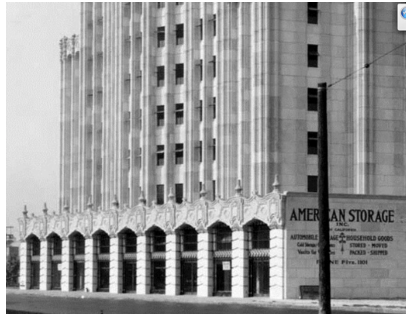
Note contrast in tone between front pillars of arcade and the rest of the faux ashlar surfaces of the building. A white stucco finish may have been applied here for aesthetic effect, perhaps similar to that detected at 710 Wilshire.
