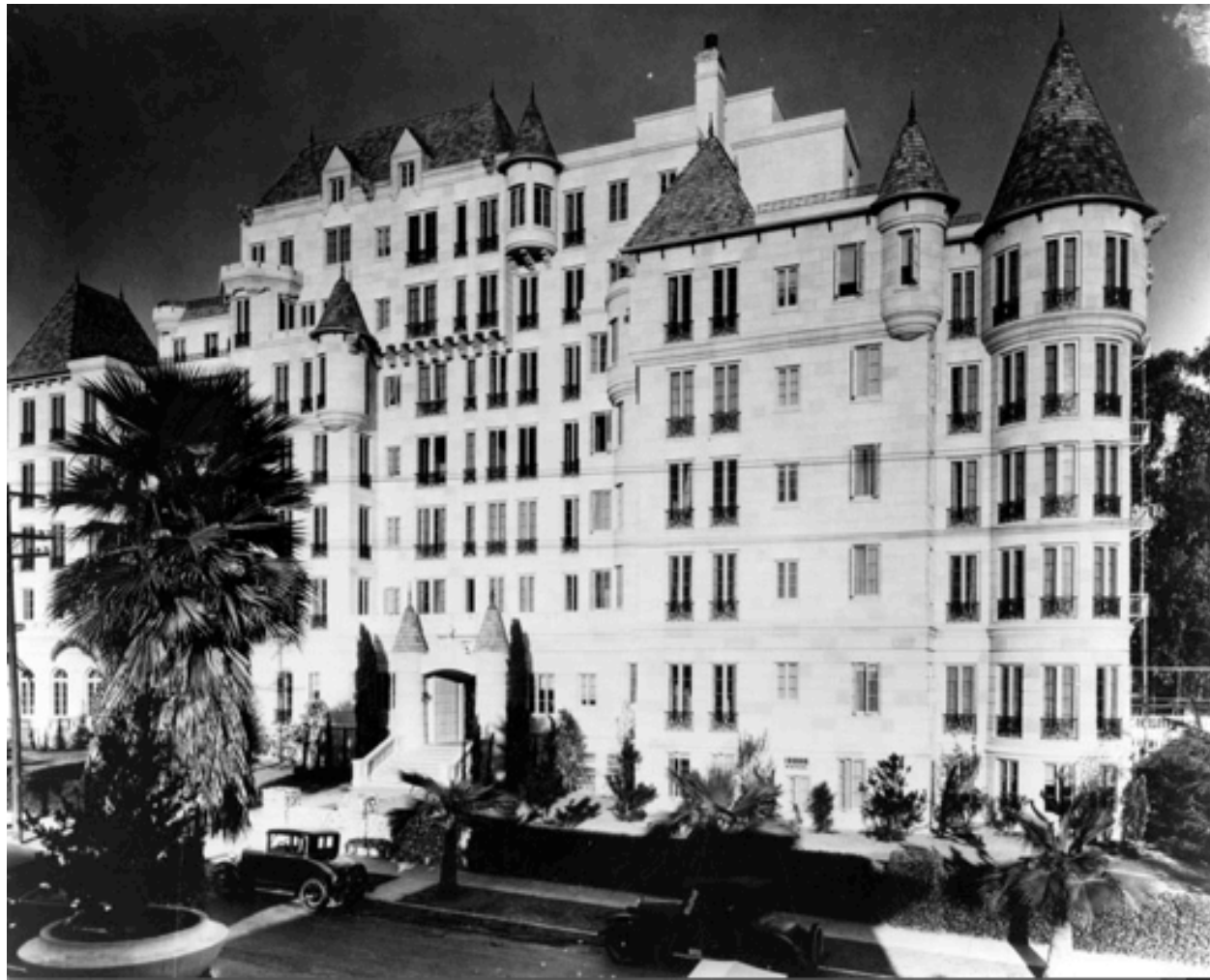
Chateau Elysee. Subtle “block” by “block” differences in tone are seen in this early photograph, enhancing the faux ashlar effect of the waste mold formed concrete. It is reasonable to assume that such aesthetic refinements may have been made at 710 Wilshire.
